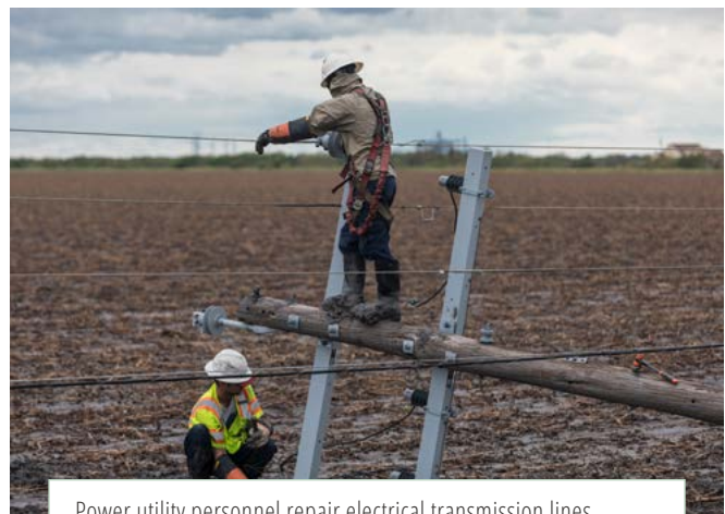
Power utility personnel repair electrical transmission lines outside the town of Rockport in response to Hurricane Harvey in Rockport, Texas, August 28, 2017. (Christopher Mardorf / FEMA.)
