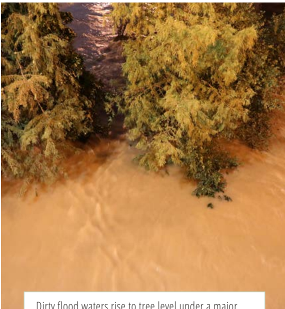
Dirty flood waters rise to tree level under a major highway bridge in Houston, Texas, August 30, 2017. (Dominick Del Vecchio/FEMA)
